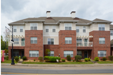
Apartment building with building articulation, including balconies.
