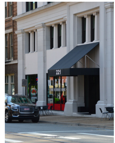
An awning is a type of appurtenance structure.
