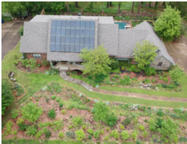
Roof-mounted solar panels. Photo: Layet Johnson
