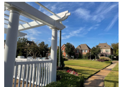
These Residential Cluster Development examples show open space and reduced lot sizes.
