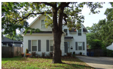
J-swing garages allow for parking in front of homes while preserving a cohesive property frontage.
