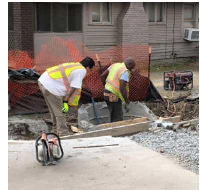
Drainage improvements under construction.
