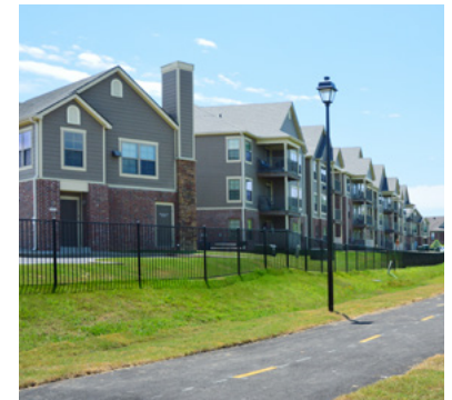
Multi-use structures facing a shared use path.
