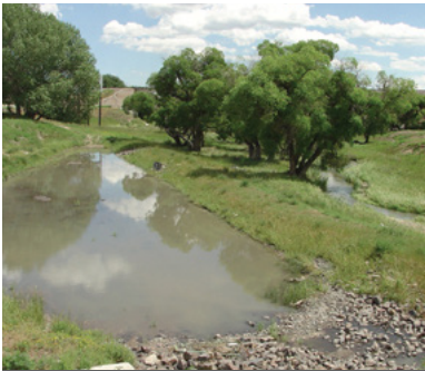
Detention ponds hold water for a short period of time; this pond temporarily holds water before it enters the stream. Photo: https://www.lccdnet.org/wp-content/uploads/Ponds.pdf
