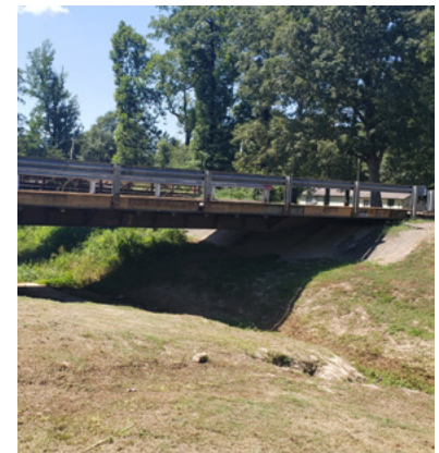
Bridge over a drainage path.
