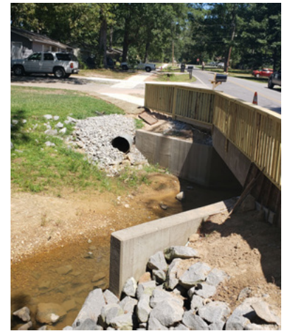
Box culvert with sidewalk.
