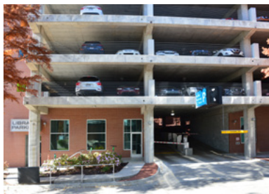
A parking deck.
