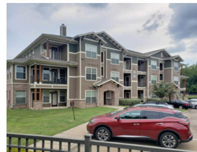
This multi-family development was constructed as a PUD on a large parcel, and includes amenities such as a swimming pool and a dog park.
