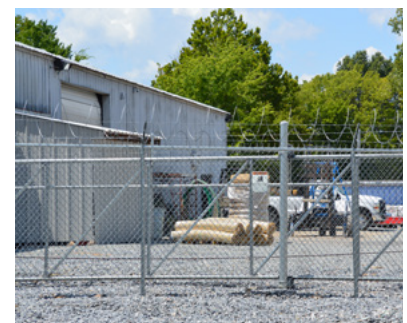
Chain-link fence with razor wire.
