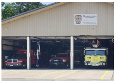
A fire station.
