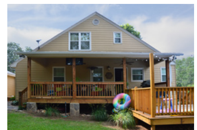
A deck attached to the principal structure.
