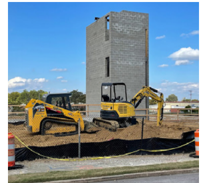
A commercial building under construction.
