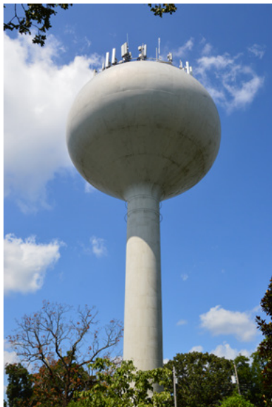
Examples of antennas attached to existing structures.
