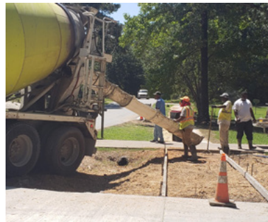
A sidewalk under construction.
