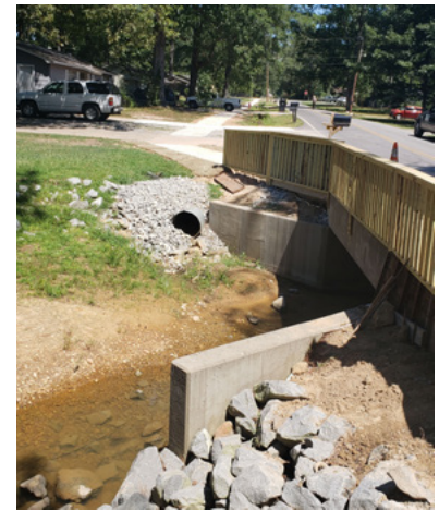
Box culvert with sidewalk.
