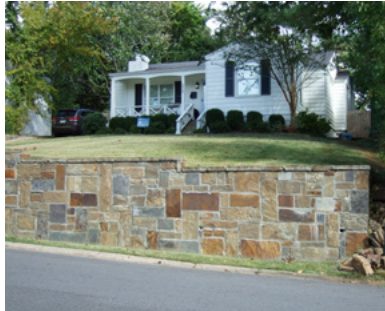
A retaining wall.
