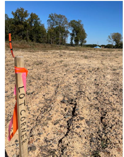
Example of a lot corner marker.
