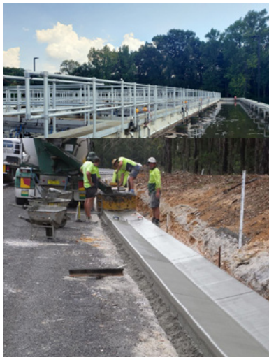
Concrete Valley. Photo: https://www.seattlewapaving.com/concrete-paving.html
