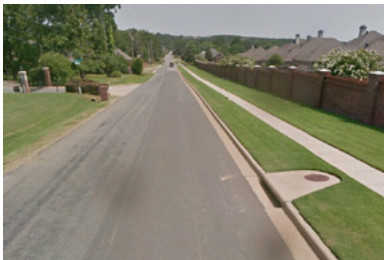
The developer of the subdivision on the right has installed half-street improvements on the boundary street per the Master Street Plan and Subdivision standards.
