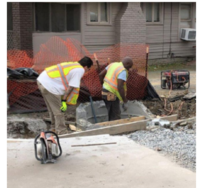
Drainage improvements under construction.
