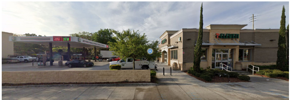
Gas canopies behind a garden wall.
