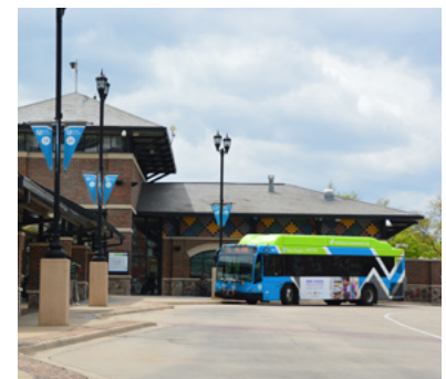
A transit terminal.
