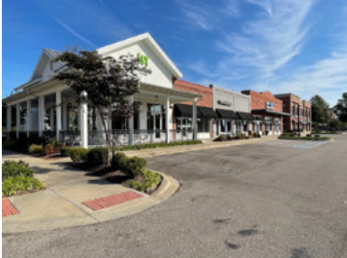
Commercial Corridor buildings with maximum front parking.
