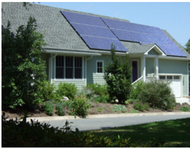
Roof mounted solar panels.
