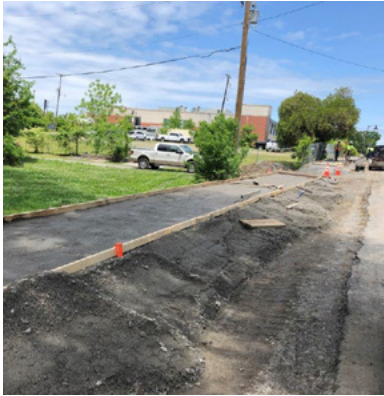
A roadway and sidewalk under construction.
