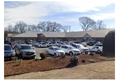
This L-shaped building has approx. 65% of its façade set back farther than the maximum setback. Photo: Google Street View.
