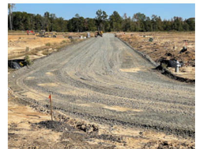
A new street under construction.
