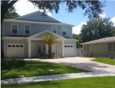
This duplex features a narrow driveway opening at the sidewalk, which then widens to accommodate two garages and additional parking. Image: Bungalower
