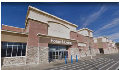
Example of a well-articulated Walmart. Source: Google Streetview.
