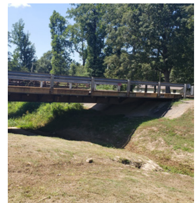
Bridge over a drainage path.
