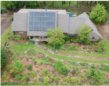
Roof-mounted solar panels. Photo: Layet Johnson
